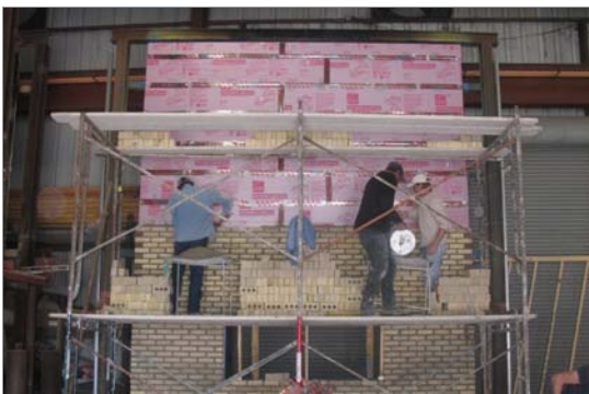
Figure 3: Test wall under construction
