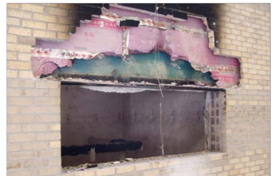
Figure 5: FOAMULAR® showing limited damage above the test window with brick veneer stripped away after the fire test
